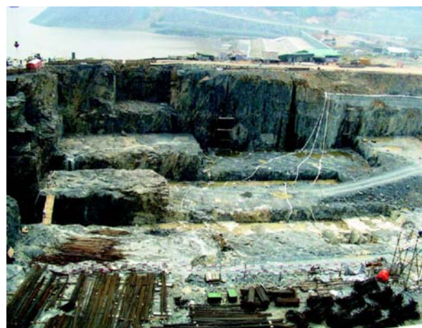
Figure1. Precision Blasting (Source: Khan, 2009)
