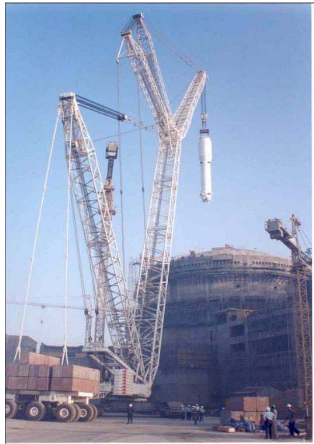
Figure 7. Steam Generator Installation in PHWR (Source: IAEA, 2004)
