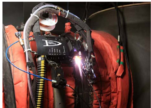
Figure 15. Automatic Welding of Reactor Coolant Pipes (Source: KEPRI, 2009)
