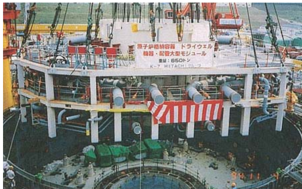
Figure 6. Open Top Construction (Source: Yahagi, 2009)
