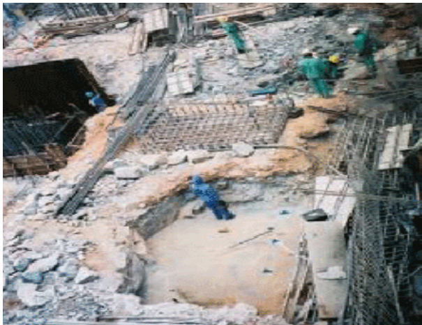
Figure 2. Excavation Using Chemical Foam Expansion (Source: IAEA, 2009)
