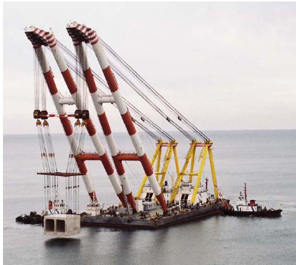
Figure13. Discharge Tunnel's Module (Source: IAEA, 2009)
