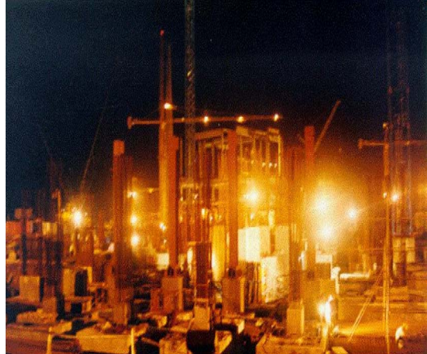
Figure 17. Night View of Construction Activities (Source: Bohra, 2006)
