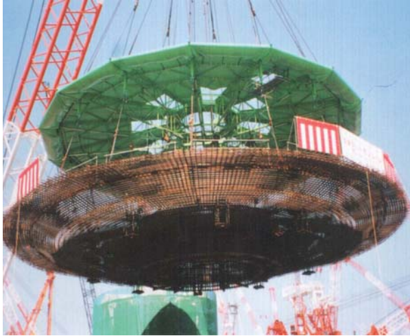
Figure 8. Base Slab Rebar Module (Source: Khan, 2009)
